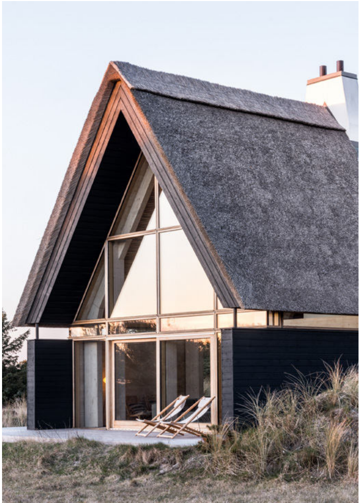
Reference: PAX architects, Skagen Klitgård
