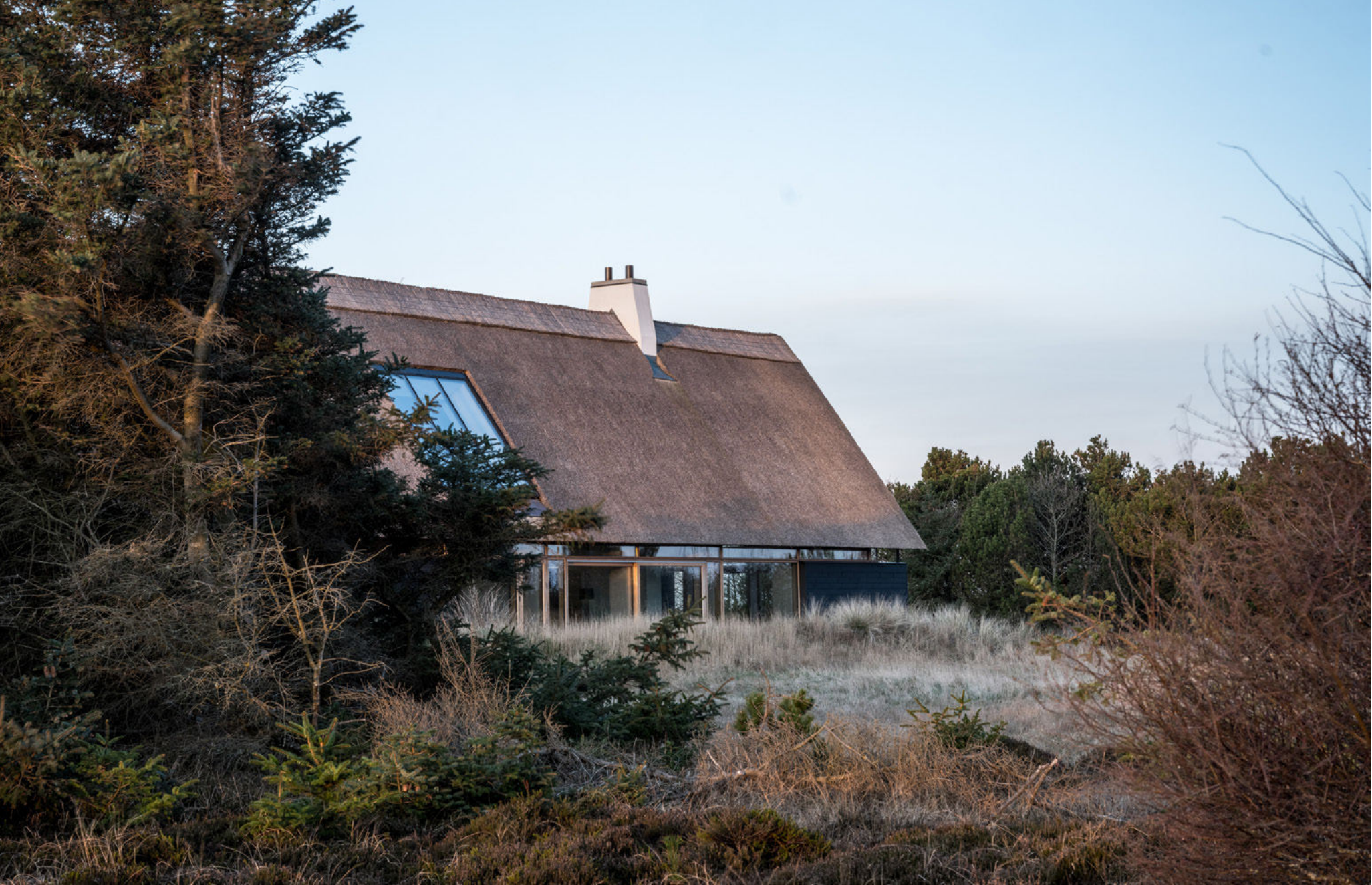
Reference: PAX architects, Skagen Klitgård
