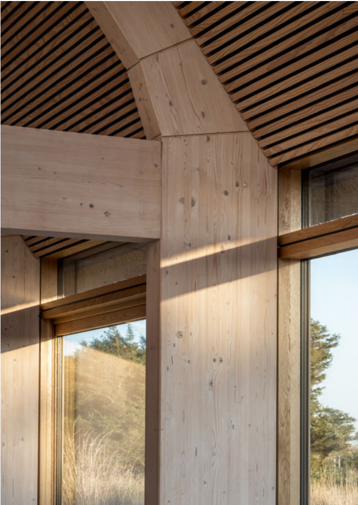
Reference: PAX architects, Skagen Klitgård
