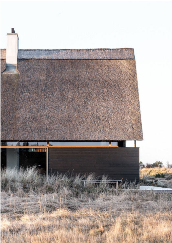
Reference: PAX architects, Skagen Klitgård
